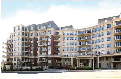
KINGSWAY CONDOMINIUMS 2855 BLOOR ST. W
