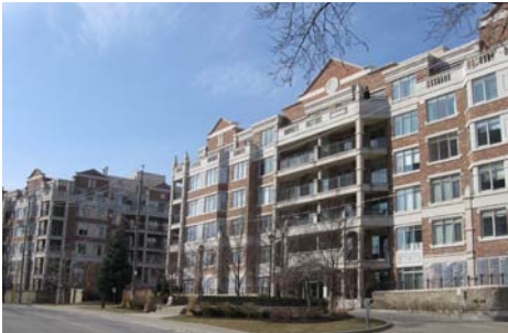
KENSINGTON I AND II 10 – 12 OLD MILL TRAIL
